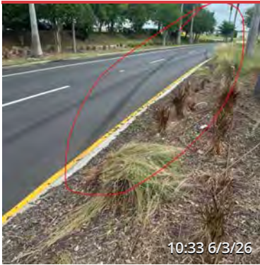
VEHICLE DROVE INTO MIDDLE ISLAND AND CAUSED SOME DAMAGE
