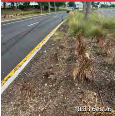
GRASSES REMOVED FROM VEHICLE DAMAGE
